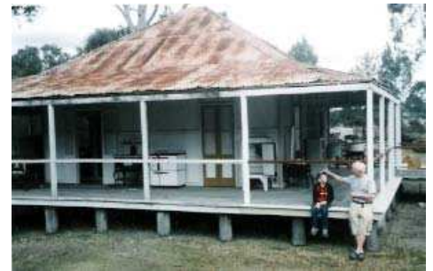
Early Queenslander (veranda & stumps help keep the occupants cool by allowing air to circulate around and under the house). Possibly mid to late 1880's
